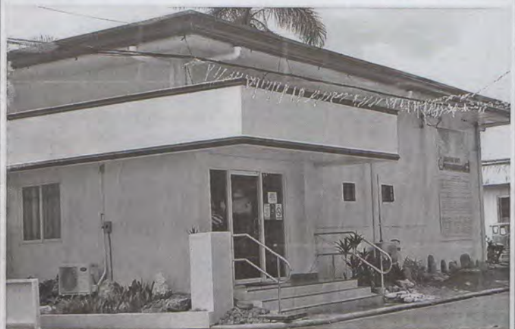
The improved Gabaldon building now houses the new Office of the President, along with Office of the BOT and Office of the Vice-Pres. for Research and Extension.
